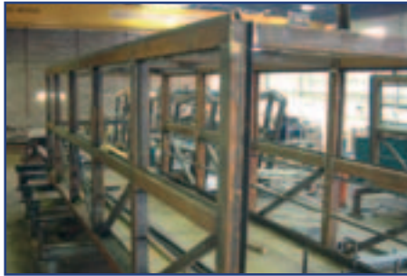
Footbridge under construction at Taylor & Sons' Cardiff workshops
